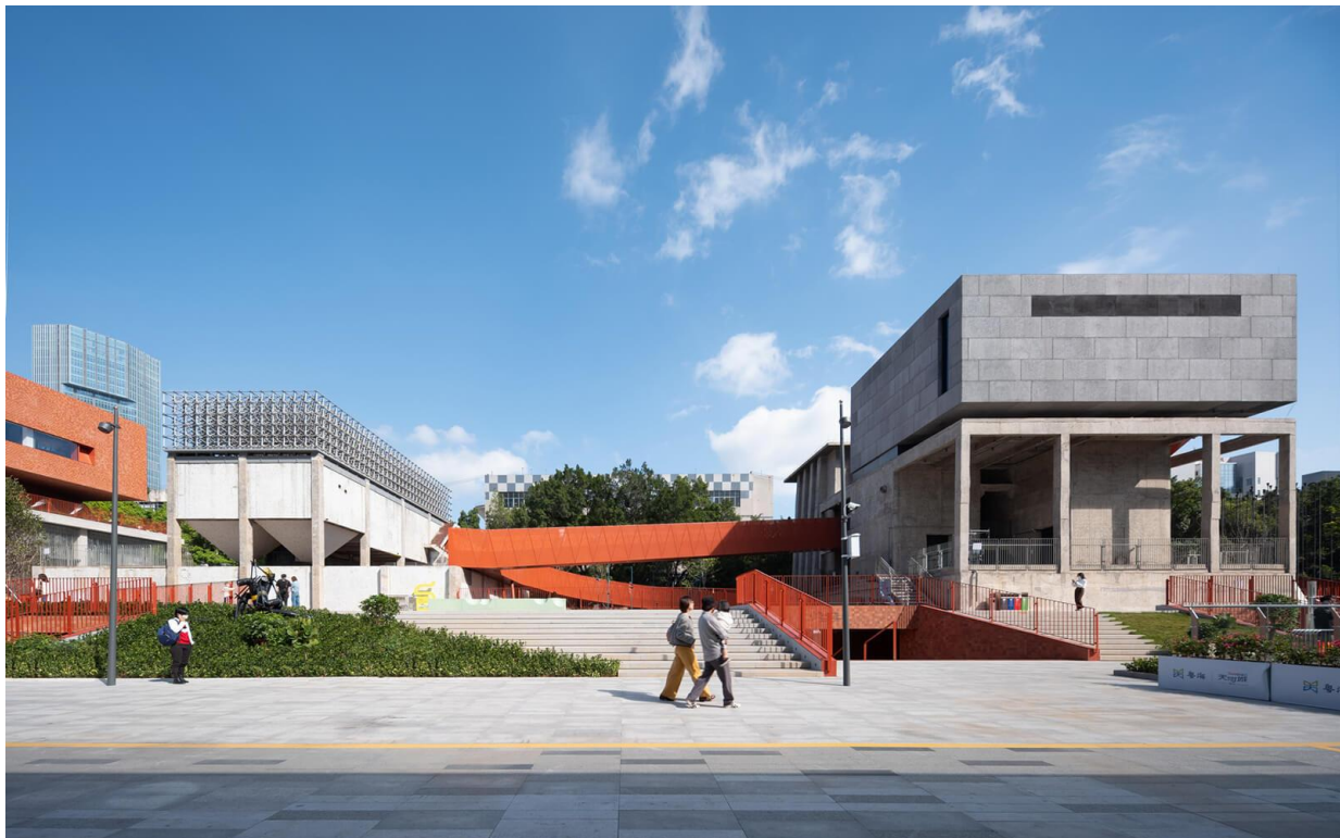
URBANUS breathes new life into the run-down structures of a former brewery in Shenzhen, China paying homage to the legacy of the site Image: © TAL
